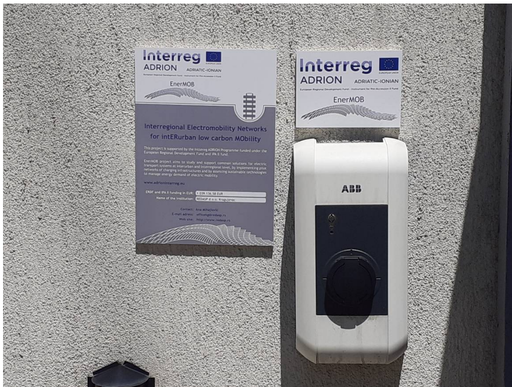
Figure 3 The private, facade electrical vehicle charger - Slow-Charging installed on the external wall of the business premises
